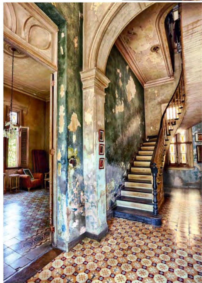
House of Fefa (stairway) – Havana
